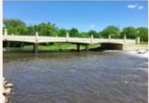
#2 THE ZUMBRO RIVER BRIDGE
