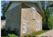
#9 SEVERANCE CARRIAGE HOUSE +
